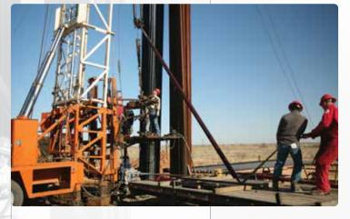
The *MetalSkin* cased-hole liner can be easily installed with a workover rig. No high-volume pumping equipment is required.
