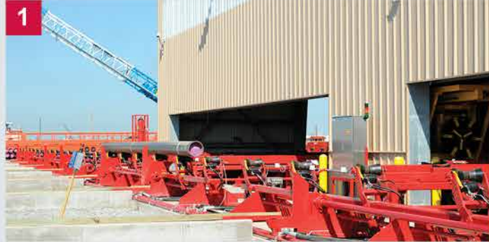
1 Pipe is loaded onto hands-free exterior conveyors and rolled inside the building. Two conveyors allow multiple pipes to be moved simultaneously.
