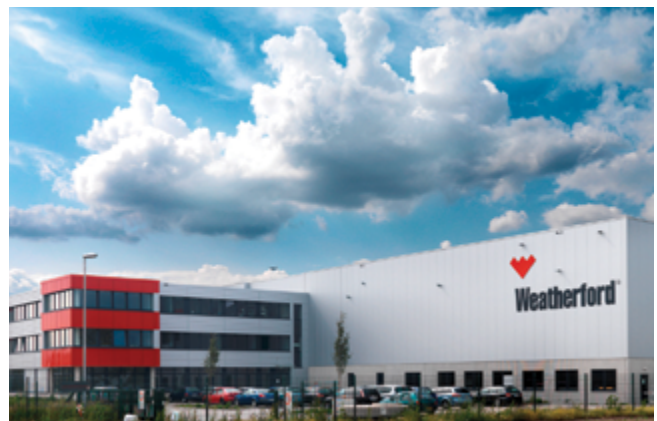
Hannover, Germany, Manufacturing Plant
