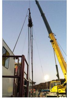
The Weatherford coiled-tubing-conveyed MetalSkin cased hole liner enabled the operator to complete fracturing operations in a short time frame in a natural gas well.
