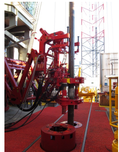
The LinkMaster tong adaptor interfaces a Weatherford power tong with a NOV ST 160 positioning device.
