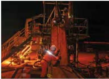
Night installation of Weatherford waterflood injection system.
