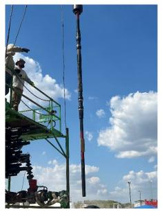
By setting cross-annular plugs from the tubing, the Reclaim solution substantially reduces the time and costs associated with pulling and properly disposing of contaminated tubing. This rigless, thru-tubing process saves valuable time and costs without sacrificing barrier performance—ensuring longterm environmental protection.
