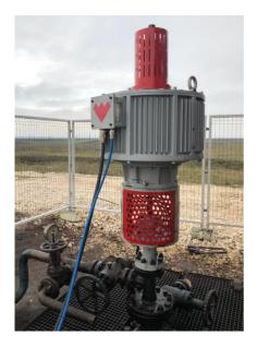
Weatherford Universal PMMs for PCP are mounted directly to the rotor, for cooler-running, lower-noise operations and reduced maintenance costs. PMMs supply up to 2,641 lbs/ft of torque at frequencies as low as 5 Hz and shaft speeds as low as 30 rpms.
