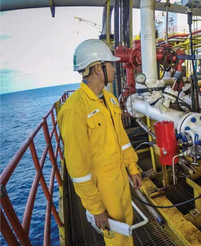
Red Eye MP water-cut meter offshore installation
